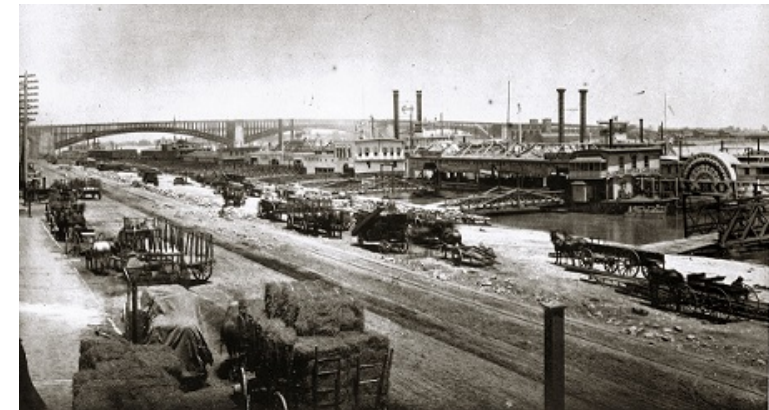
St. Louis Riverfront Levee
