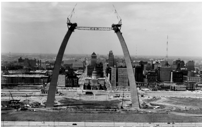
Building of the Gateway Arch
